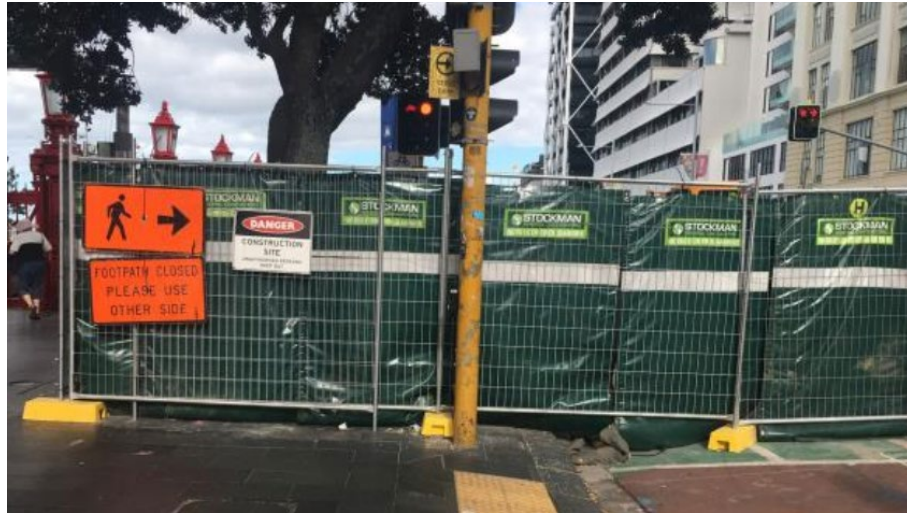
Figure 2 – Typical 1.8m site fencing with sound blanket/ barrier (as required) for short term establishments with moderate works.
