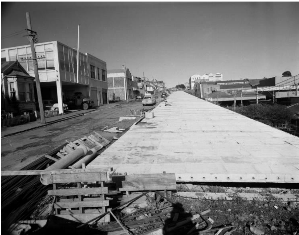
Figure 16. Photo, dated 1956, facing south showing the street widening project in Nelson Street, Auckland, nearing completion (source: Auckland Libraries Heritage Collections 580-02199)
