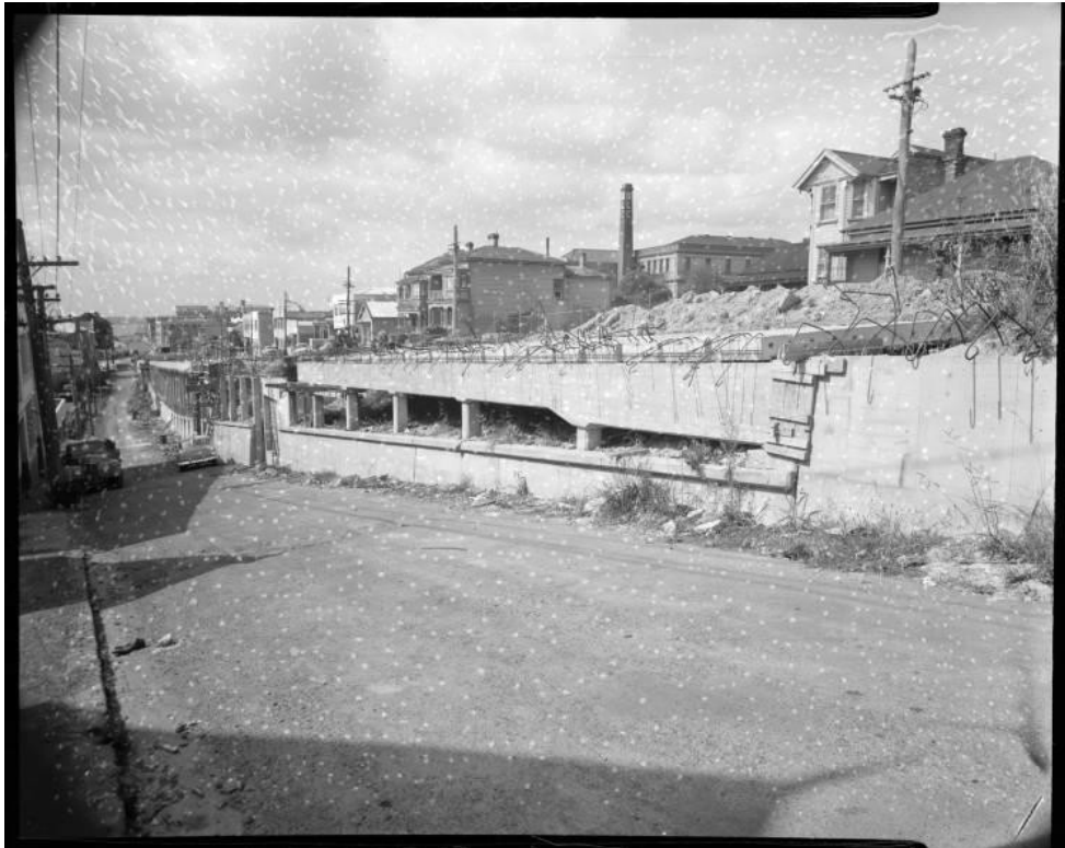
Figure 15. Photo facing northeast showing the viaduct on the newly widened Nelson Street, dated 1956 (source: Auckland Libraries Heritage Collections 580-02041)
