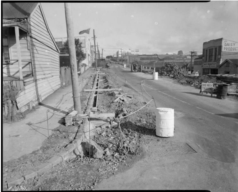
Figure 13. Photo, dated 1954, facing south showing the kerbing construction on the eastern side of Nelson Street (source: Auckland Libraries Heritage Collections 580-01410)
