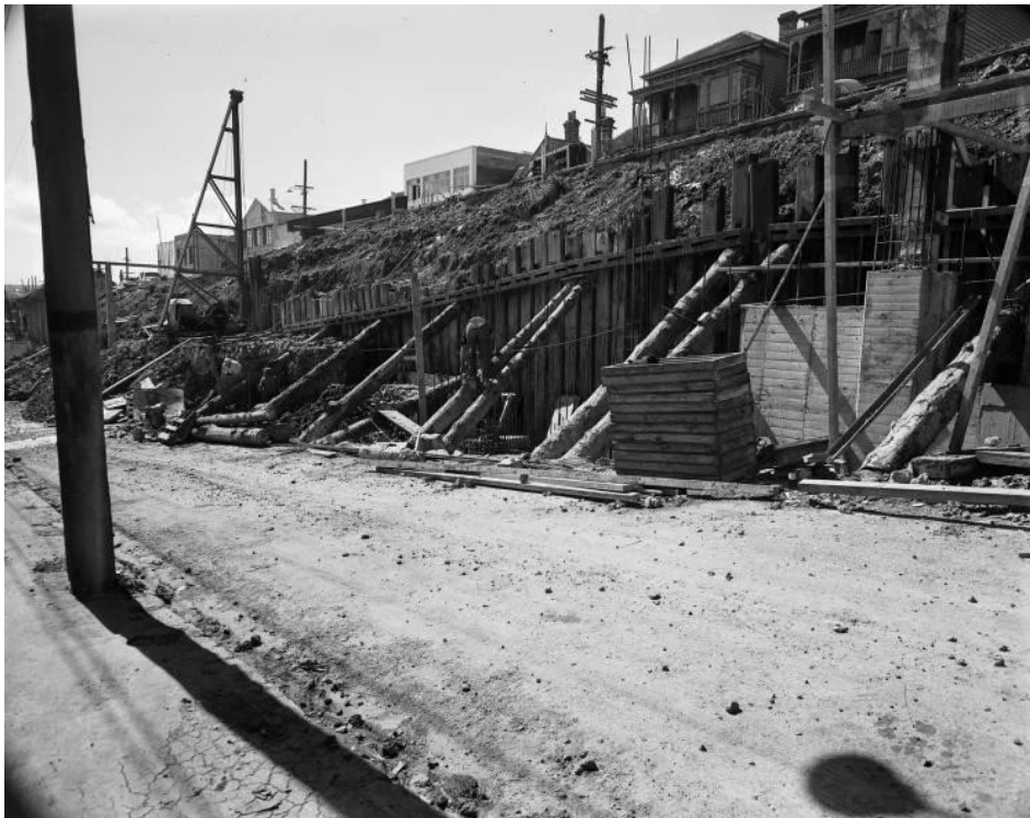
Figure 14. Photo, dated 1955, looking northeast, showing the construction of a temporary retaining wall for the viaduct during the widening of Nelson Street (source: Auckland Libraries Heritage Collections 580-01757)
