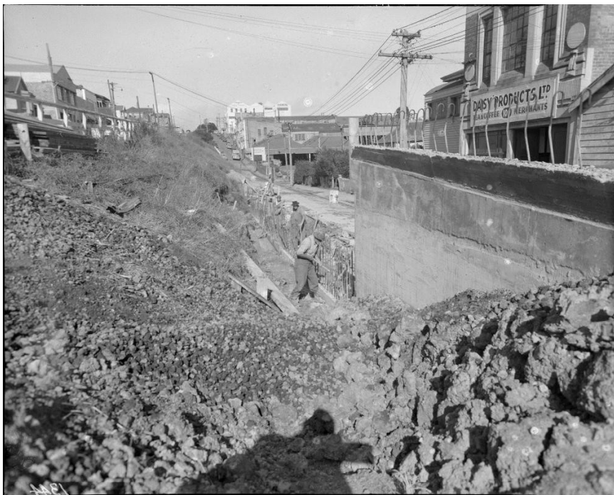
Figure 12. Photograph, dated 1954, with a view facing southwest, showing the construction of a retaining wall during the widening of Nelson Street (source: Auckland Libraries Heritage Collections 580-01344)
